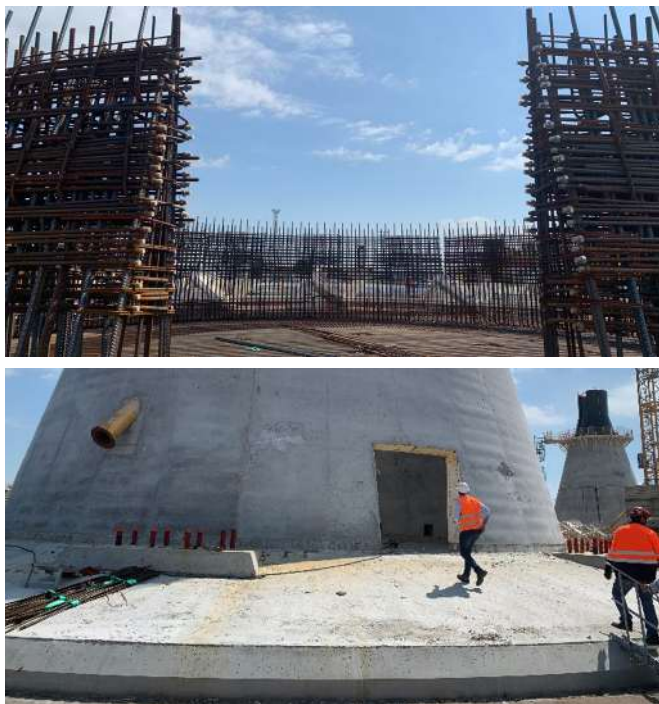
Use of couplers for “clean” wall openings avoiding protruding rebars
