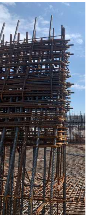
Use of couplers for “clean” wall openings avoiding protruding rebars
