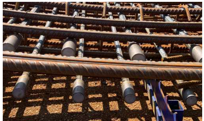
Walls starter bars connected
