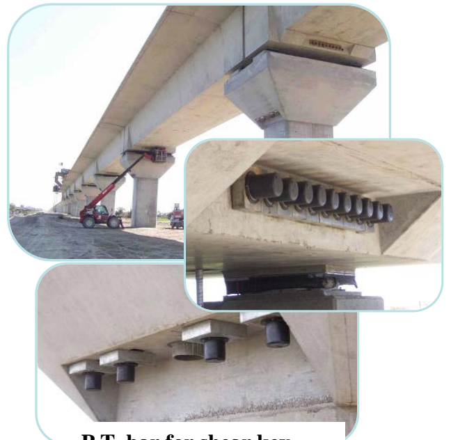
P.T. bar for shear key
