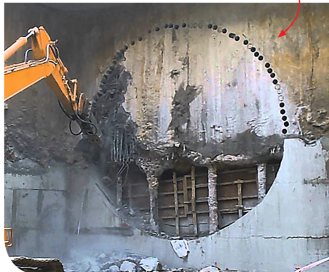
Removal of concrete and steel structure
