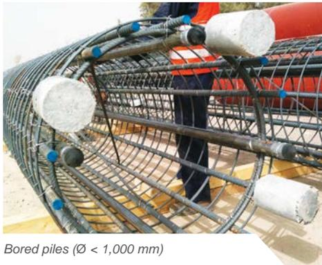
Bored piles ( $\varnothing < 1,000$  mm)
