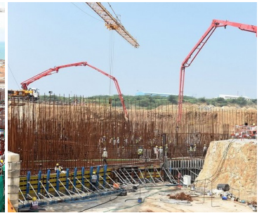
Kudan Kulam 5&6, India 2021-ongoing
