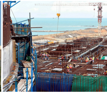
Kudan Kulam 3&4, India 2019-ongoing
