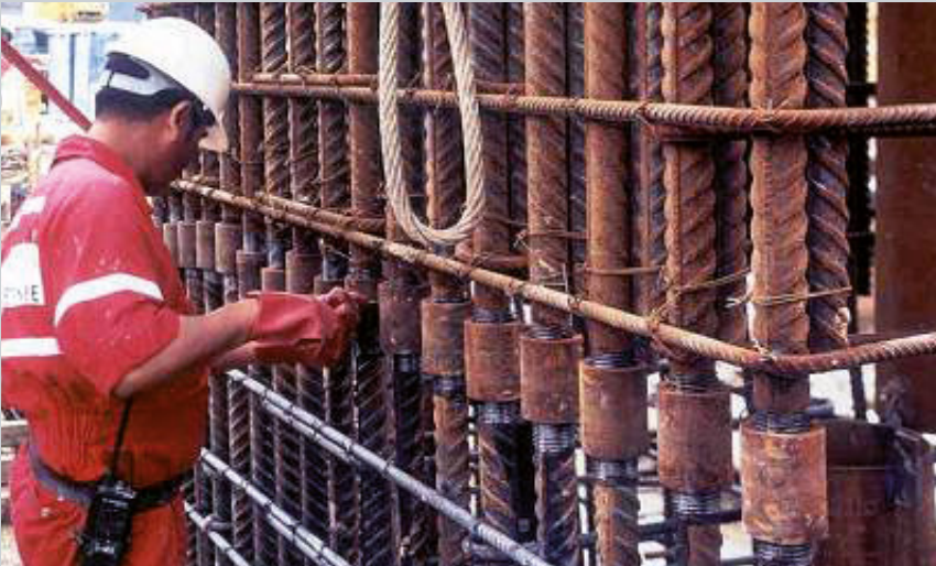
Bartec/Fortec couplers in diaphragm wall
