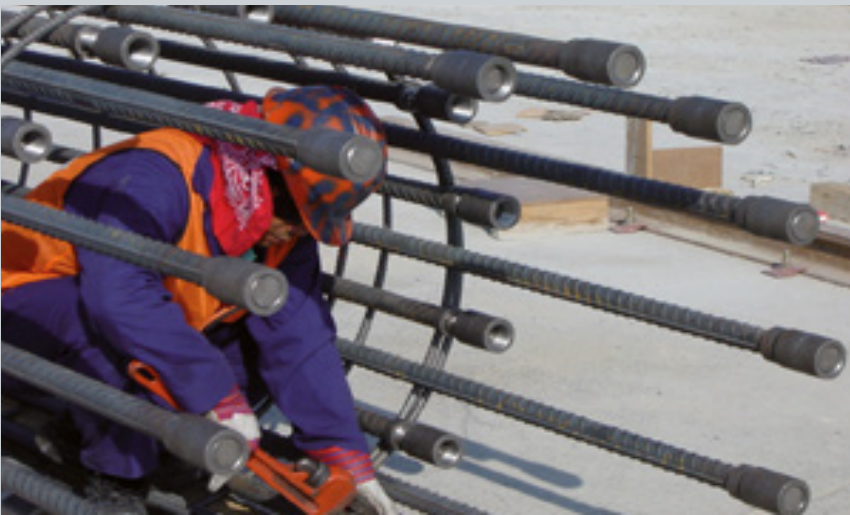
Bartec/Fortec couplers in pile cages
