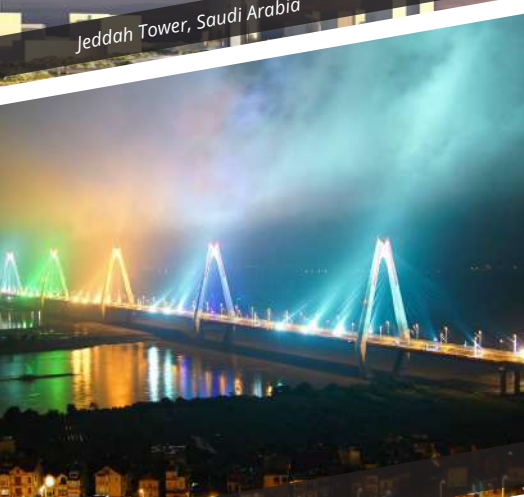
Nhat Tan Bridge, Vietnam
