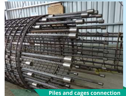
Piles and cages connection
