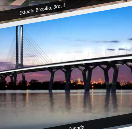
New Champlain Bridge, Canada
