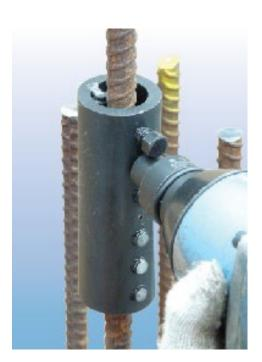
Insert the second bar into the coupler until contact with the center pin and repeat the operation. Check the bar alignment when tightening the screws with a wrench: at a distance of 25cm the misalignment should not exceed 5mm (or not more than 1/4" at a distance of 1ft).
