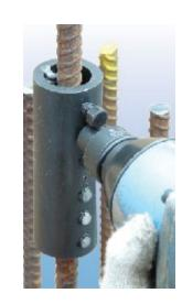
Tighten all screws, from centre to outside, with an impact wrench until their heads shear off. (A manual wrench can be sufficient for small quantities).
