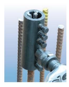
Insert the Unitec coupler over the end of the first bar until contact with the centre pin. Strongly hand tighten the screws from centre to outside with a wrench to pre-position the coupler progressively in order to maintain its alignment with the bar.
