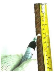
Mark the bar engagement length on each bar end, using the data in the table.
