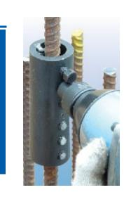
Tighten all screws, from centre to outside, with an impact wrench until their heads shear off. (A manual wrench can be sufficient for small quantities).
