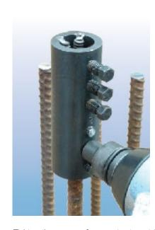
Tighten the screws, from centre to outside, with an impact wrench until their heads shear off. (A manual wrench can be sufficient for small quantities).
