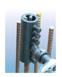
Insert the Unitec coupler over the end of the first bar until contact with the centre pin. Strongly hand tighten the bolts from centre to outside with a wrench to preposition the coupler progressively in order to maintain its alignment with the bar.
