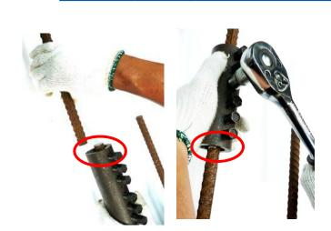
Slide the Unitec coupler over the first bar. Bring the continuation bar in front of it and slide the Unitec coupler back over it. Position the coupler between the marks and hand tighten the bolts.
