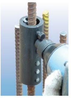
Insert the second bar into the coupler until contact with the center pin and repeat the operation. Check the bar alignment when tightening the bolts with a wrench : at a distance of 25cm the misalignment should not exceed 5mm (or not more than 1/4" at a distance of 1ft).
