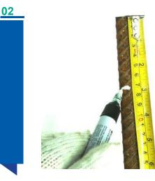
Mark the bar engagement length on each bar end, using the data in the table.
