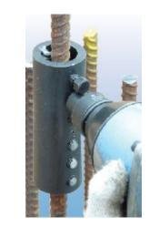
Tighten all bolts, from center to outside, with an impact wrench until their heads shear off.
