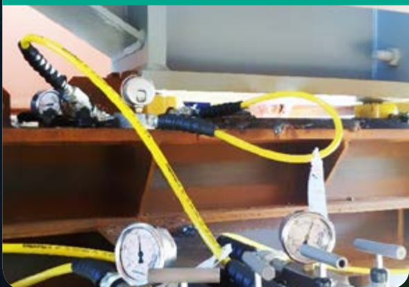
Jacking / Shimming
