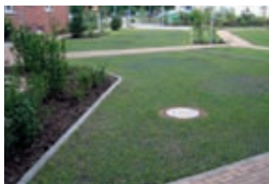
ACO grass grid used as large-scale reinforcement of fire rescue access route
