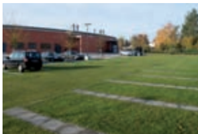
Parking space reinforced with grass grid
