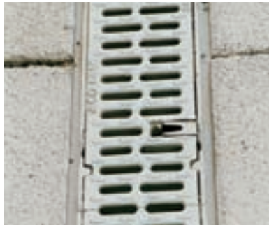
In this example, the grates and edge rails were coated grey to match the colour of the paving stones
