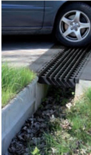
As they make their way along the ACO guide system, animals are guided under access roads without hindrance thanks to the use of stop channels.
