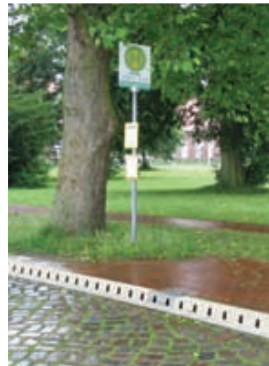
Kerbstone and drain in one, ACO DRAIN® KerbDrain
