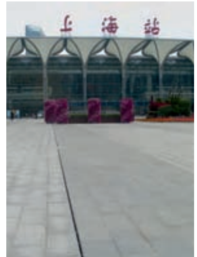
Shanghai central station. The slot can be offset in harmony with the architectural design of the surface
