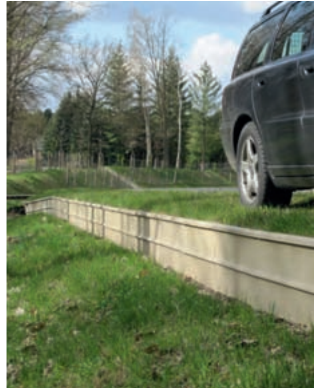
As they make their way along the ACO guide system, animals are guided under access roads without hindrance thanks to the use of stop channels.
