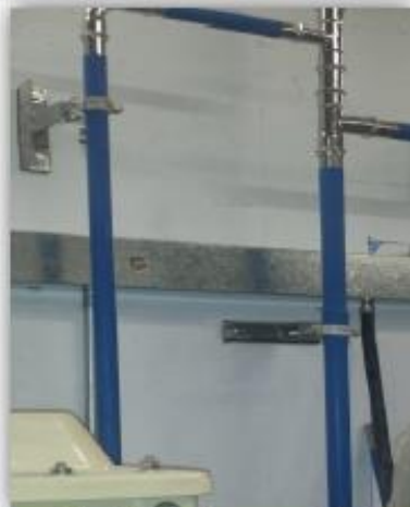
Installed by Electrical Tools
