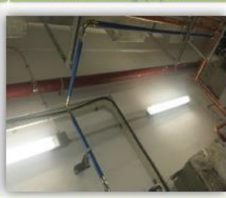
Installed by Electrical Tool
