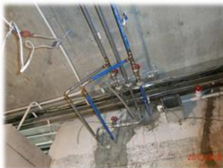
Installed and in connection with Valves
