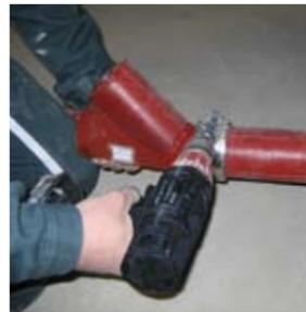
Cast iron wastewater systems are installed using simple tools eg ratchet, spanners and does not use glue or solvents, which could be harmful to installers' health.
