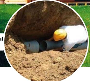
Pipe System for Horizontal Ground-Coupled MV
