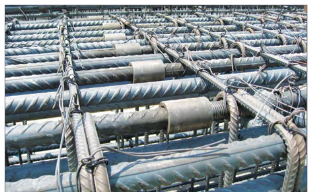
Figure 2. The use of rebar couplers can reduce rebar congestion as it eliminates the requirement to lap rebar.
